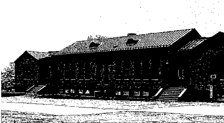
Fox Middle School – New Roof and Exterior Improvements
