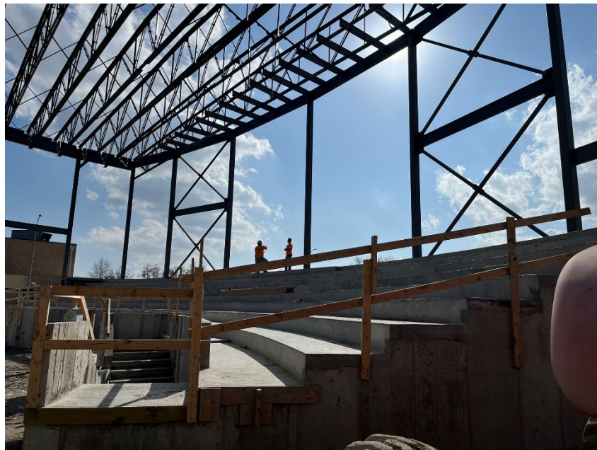
Kirkville School District – New Performing Arts Center under construction
