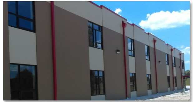
New Linn Elementary School – Classroom Wing
