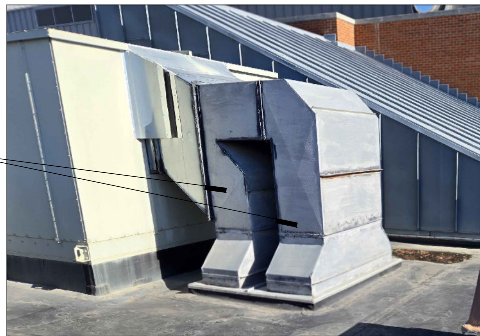
7 PHOTOS OF EXISTING DUCT WORK TO BE COVERED IN ROOFING MEMBRANE A-3 NTS
