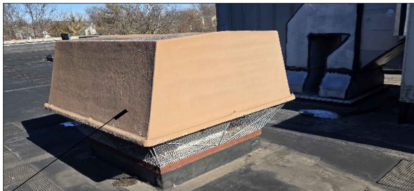
REPLACE ENTIRE VENT ASSEMBLY PROVIDING SAME FUNCTION, FABRICATE IN SHEET METAL. DESIGN TO PREVENT WATER INFILTRATION. USE RUST-RESISTANT MATERIALS.
