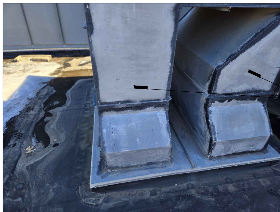
7 PHOTOS OF EXISTING DUCT WORK TO BE COVERED IN ROOFING MEMBRANE A-3 NTS
